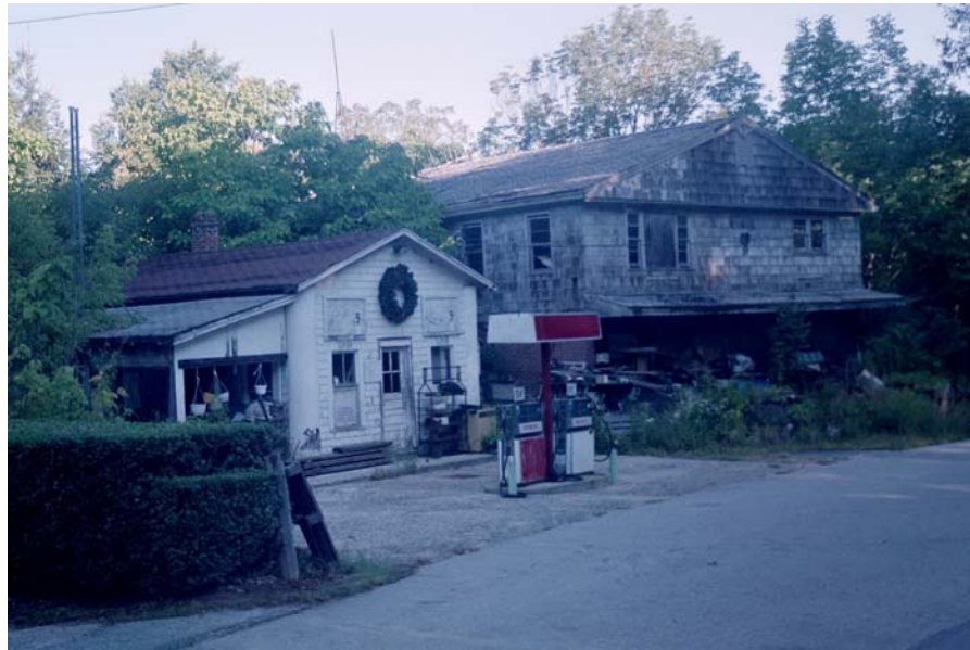
Figure 41. Old Store in Disrepair Just Off Route 12
