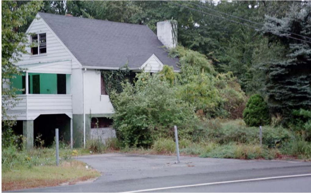
Figure 3. Boarded House along lower Route 12
